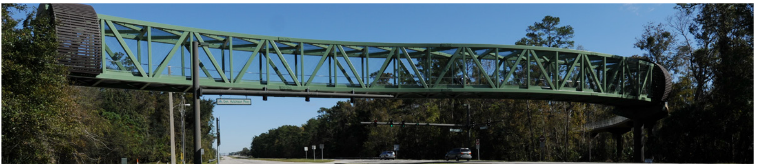
Pedestrian Bridge in Seminole County
